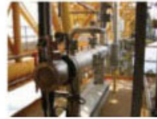
Natural gas over heater Drilling platform 100 kW Flange : 12"
