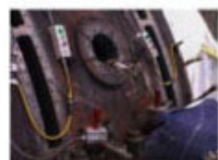
Use of bolt heaters Equipment for turbines Energy production plant
