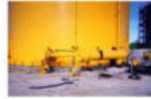
Circulation heater 500 kW, ATEX Fuel oil heating Flange : 24"
